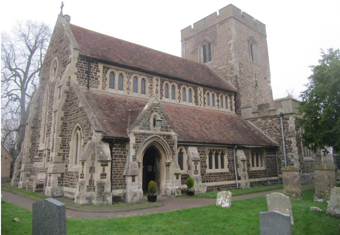
[Meppershall, St Mary the Virgin. General view from the south-west.]
